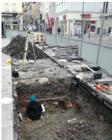
Fosse de plantation, place Grenette, Grenoble
